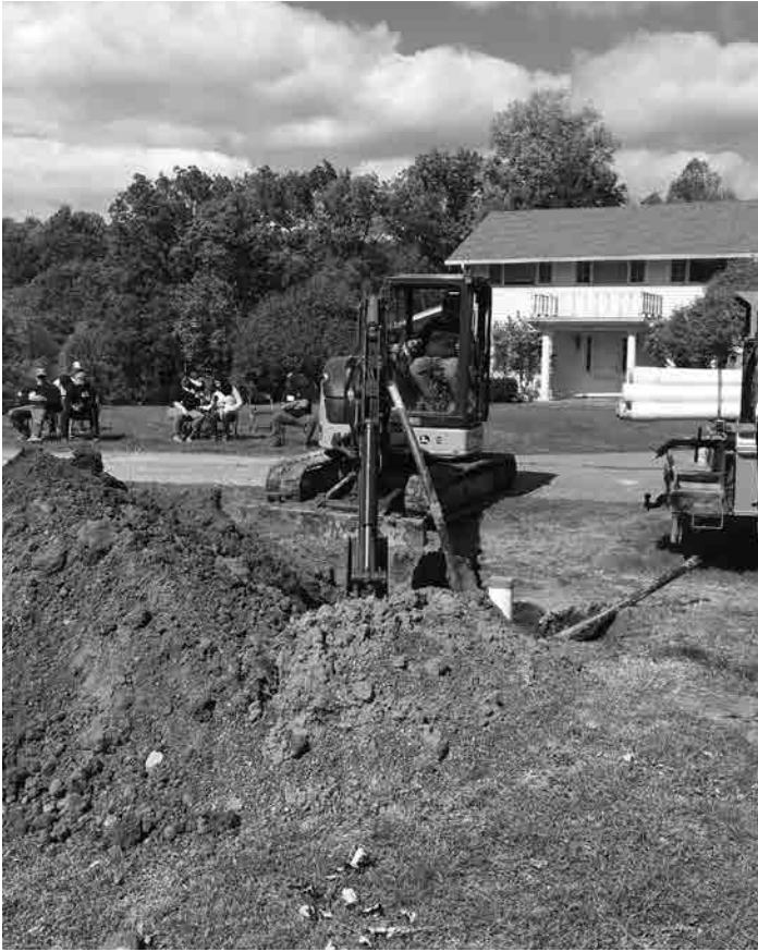
Digging up well to connect waterline.
