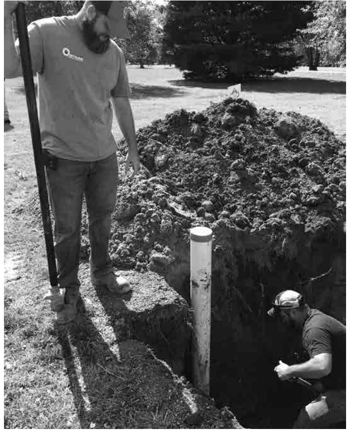
Installing outside pitless adapter.
